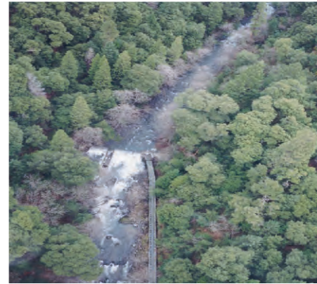
NORTH BATTLE CREEK FEEDER DIVERSION DAM
