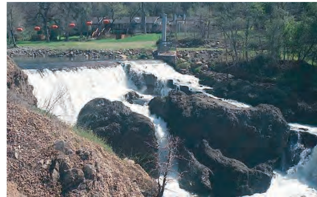
INSKIP DIVERSION DAM
