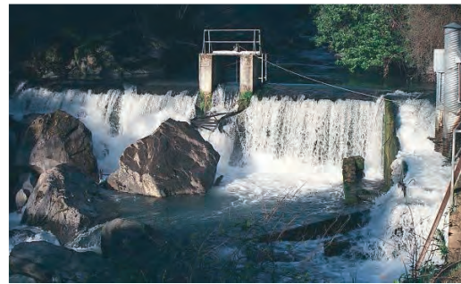
EAGLE CANYON DIVERSION DAM
