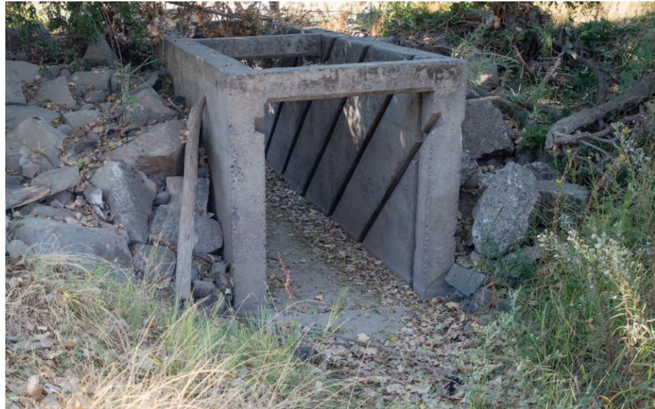
The old fish ladder at the Fremont Weir on the Sacramento River at the Yolo Bypass. There are plans to modify the 2-mile weir so it is more suitable for fish habitat.
