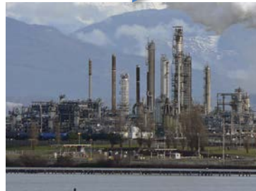
High-Pressure Boilers (RO)
