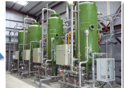
Low-Pressure Boilers (RO)
