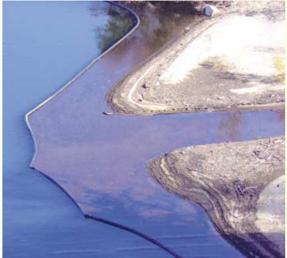
A turbidity curtain holds back sediment washed from fire-ravaged slopes into the Poway Reservoir after a rainfall.
