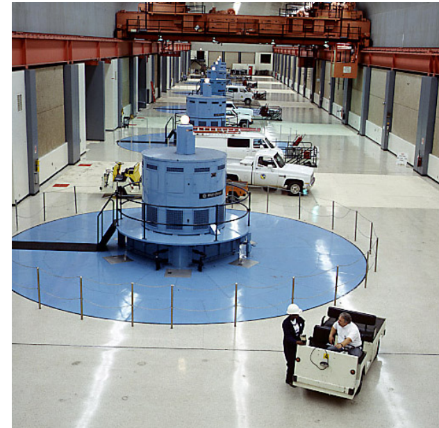
Hyatt Powerplant below Lake Oroville is in a cavern the size of two football fields.
