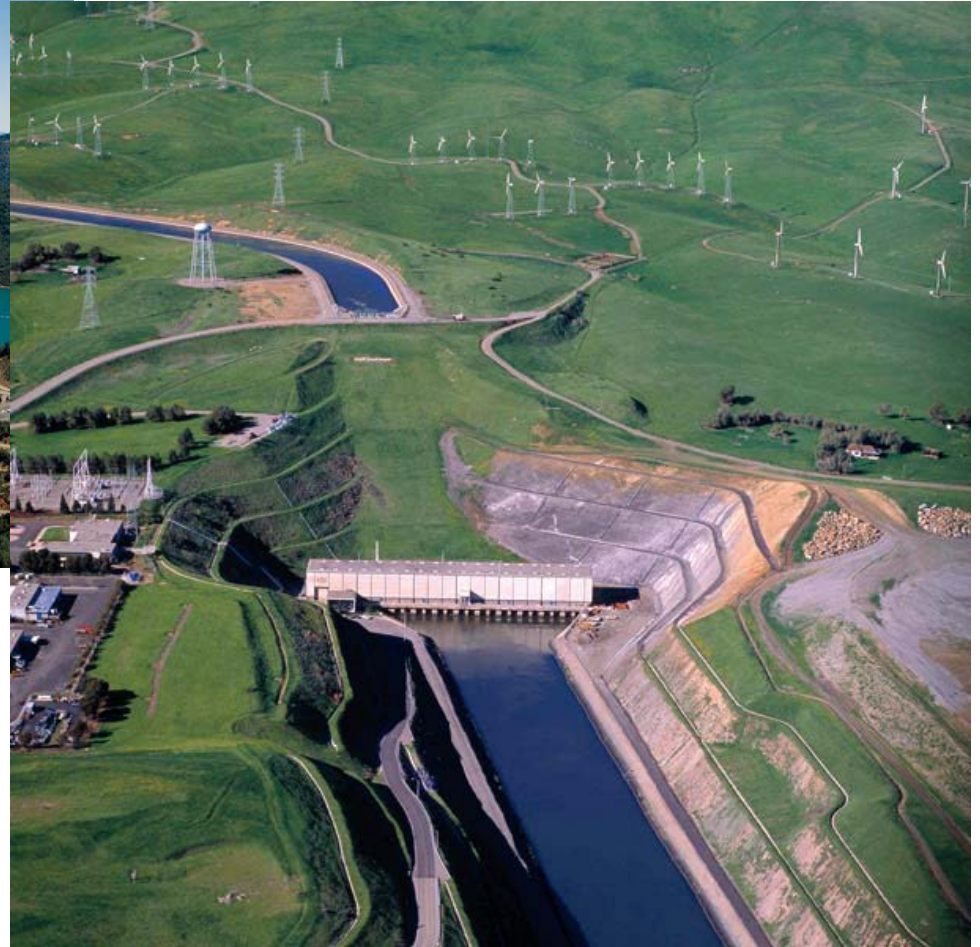
Top of California Aqueduct
