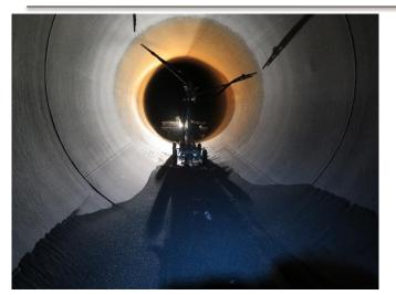
The original coal tar enamel coating in the discharge manifolds and pipes at Mark Wilmer Pumping Plant were failing. Large sheets of the enamel had completely disbonded from the primer coat. Although much of the primer coat was still intact, there were cracks throughout forming corrosion lines in the substrate.
