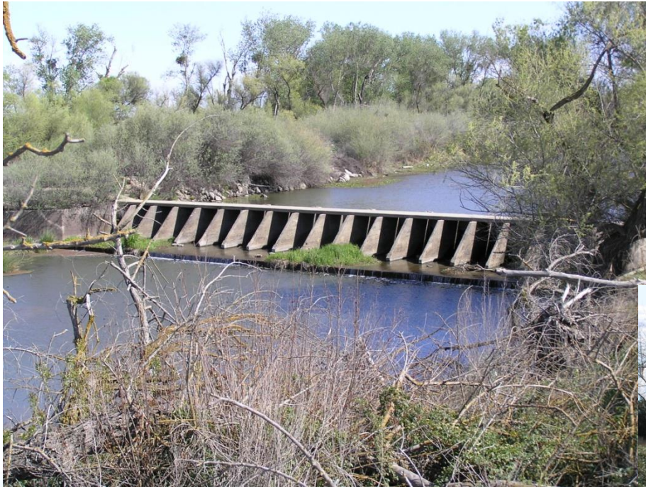
Sack Dam – Modify for fish passage
