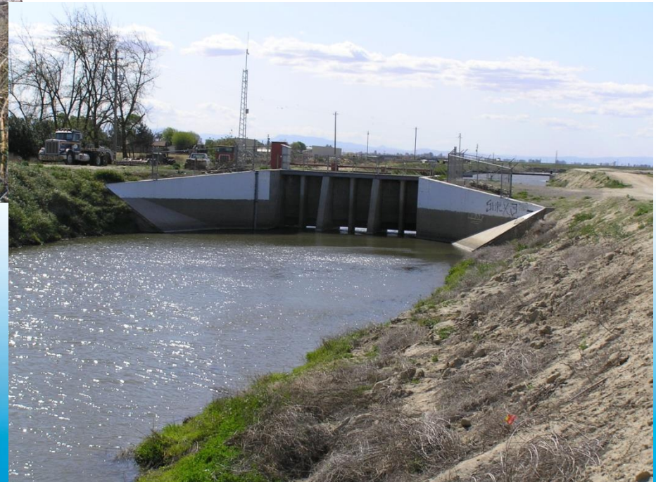
Arroyo Canal – Screen to prevent fish entrainment
