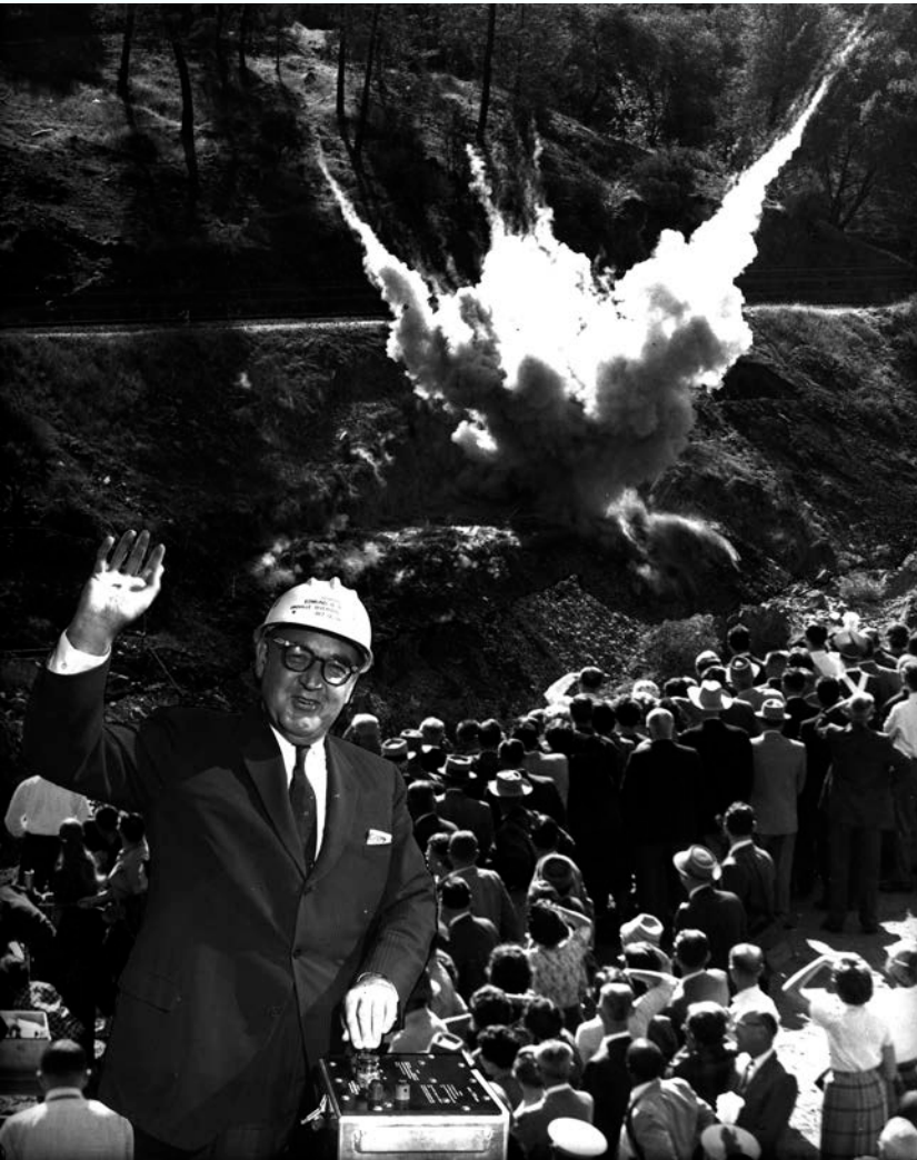
Gov. Pat Brown at Oroville Dam
