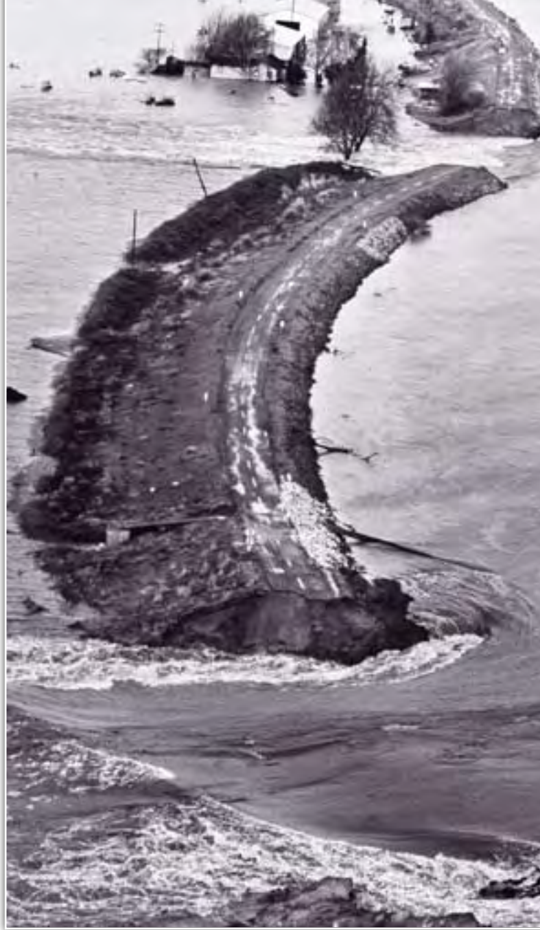
Top Photo: Levee failure in the Sacramento-San Joaquin Delta's Tyler Island during the 1986 Flood.
