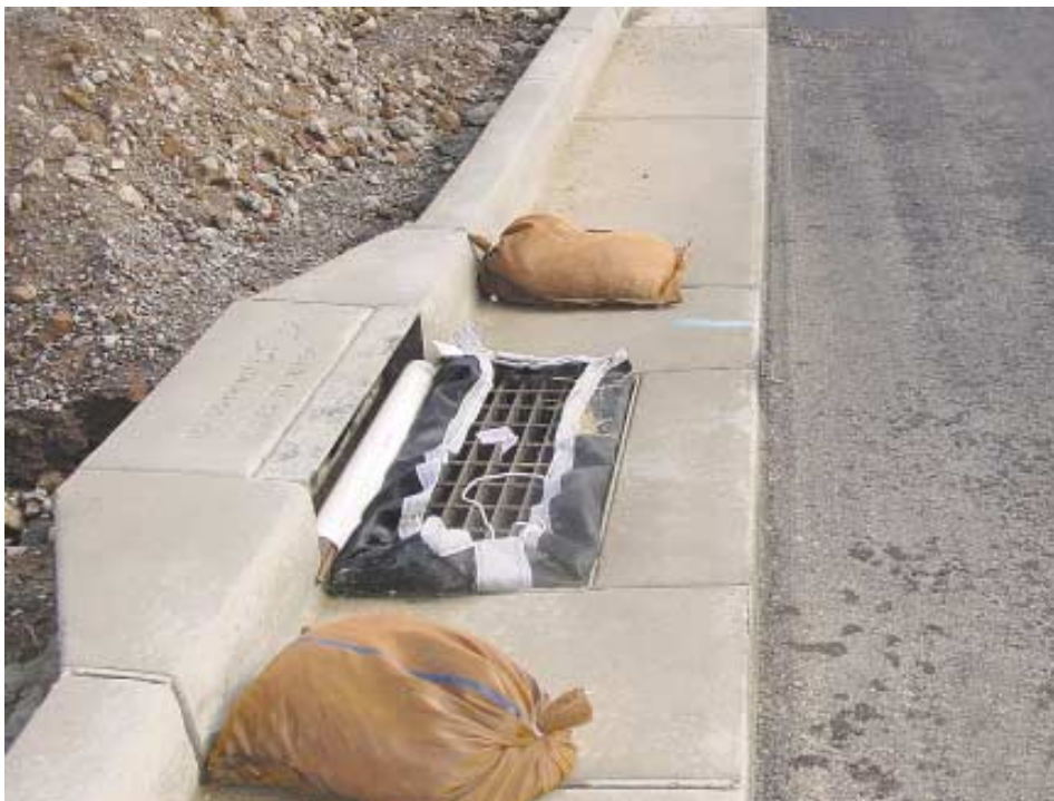
A protected drain inlet uses gravel bags and an internal filter bag to trap sediment.
