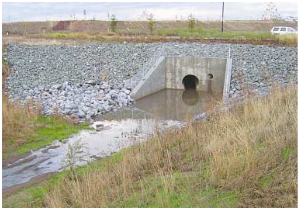
Builder improvements show culvert with clean water.
