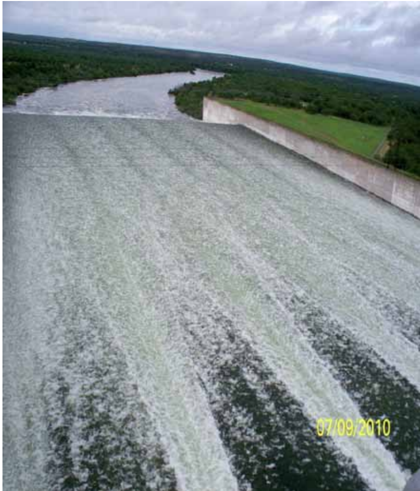
Falcon Dam view from
