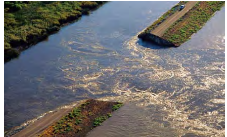
Levee Break, Roadway Washout
