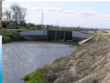
Arroyo Canal – Screen to prevent fish entrainment
