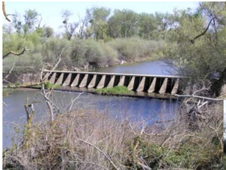
Sack Dam – Modify for fish passage
