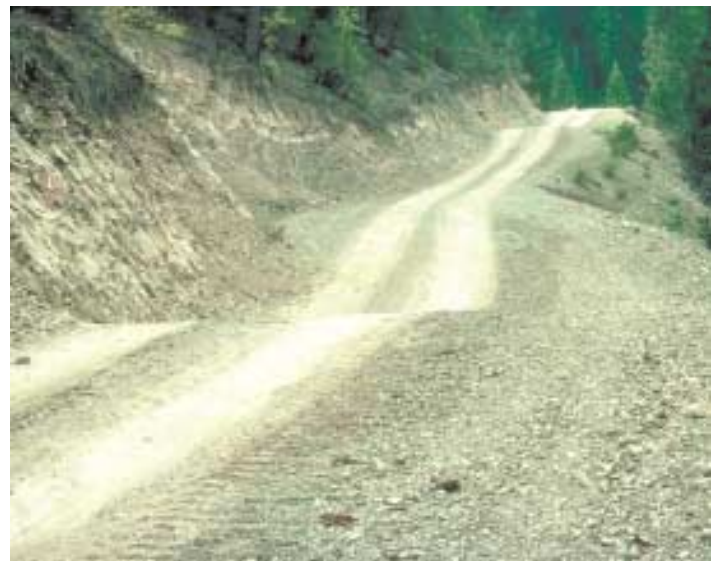
Old, rutted roads send storm water directly into streams. New road designs that protect forest water quality slope outward with rolling dips sending dispersed runoff to the forest floor.
