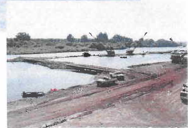
In-river construction using longitudinal berm
