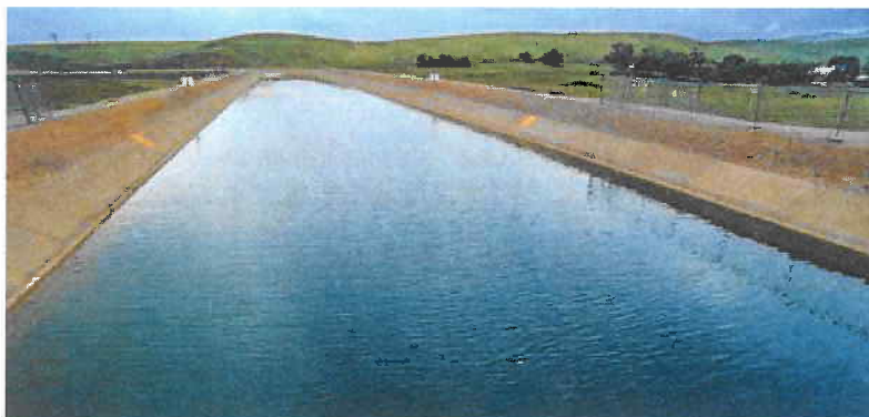
NODOS would take advantage of existing water facilities, including Tehama-Colusa Canal, as shown here.
