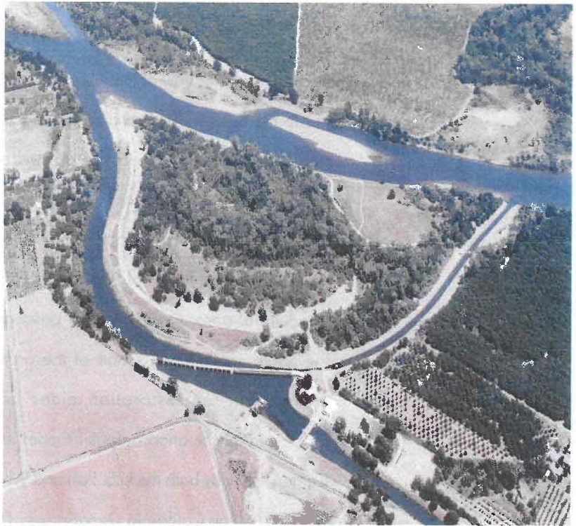
Aerial photo of the District facilities
