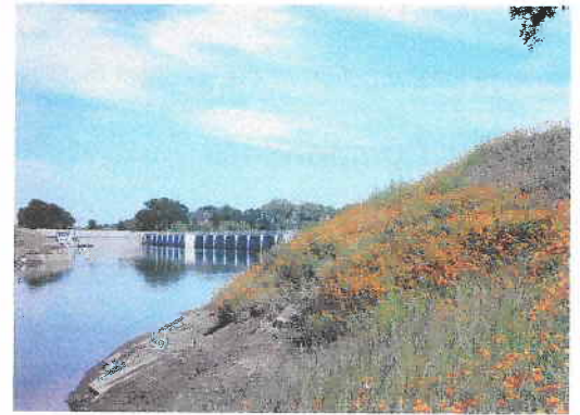
View of poppies in pump station forebay; fish screen in background
