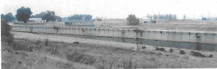
View of fish screen facility from Montgomery Island
