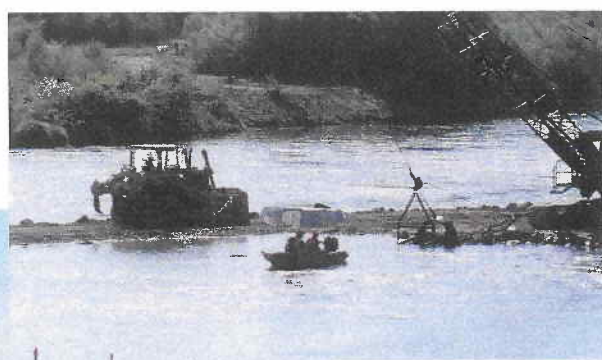
In-river construction using drag line
